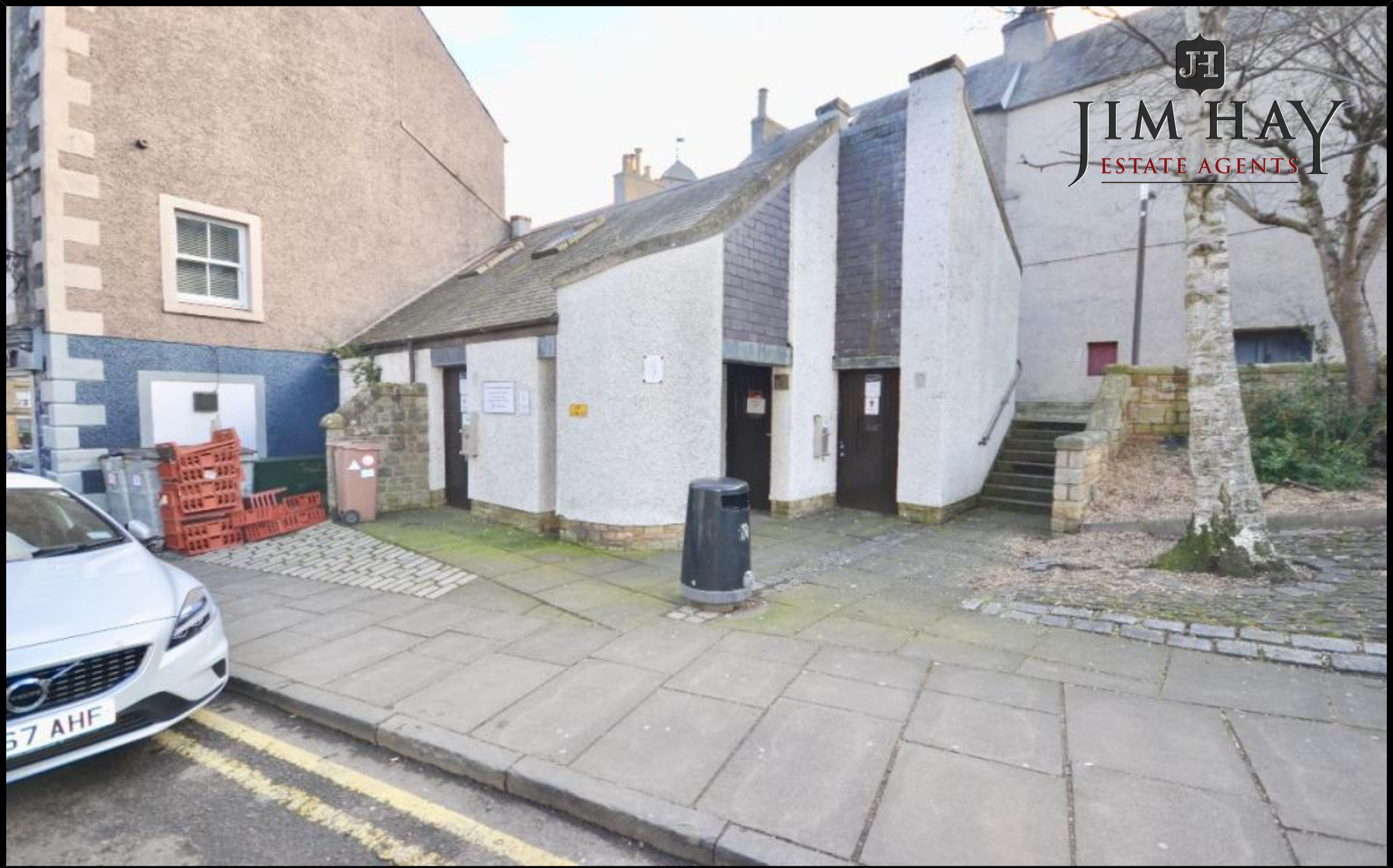
Toilet Block Howegate Hawick TD9 0AA
